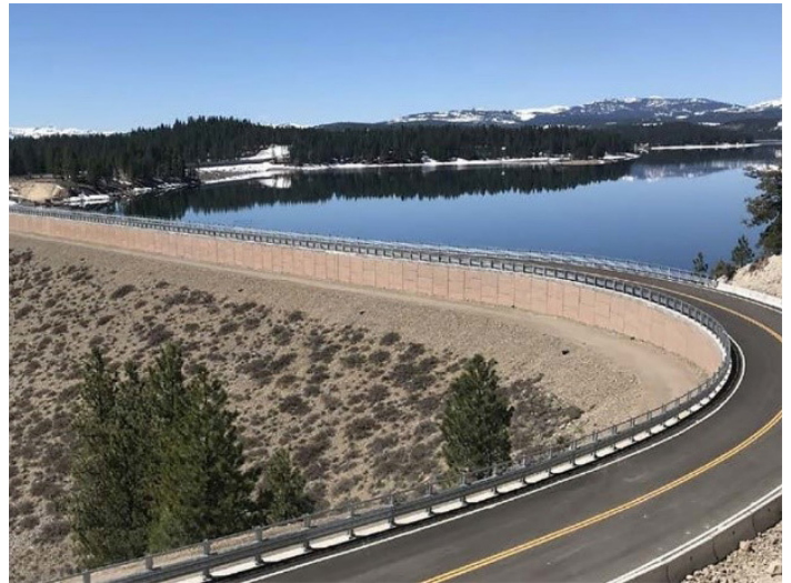
The end result of the 2018 Safety of Dams Modification Project, which strengthened the dam's embankment and raised the dam crest by 11.5 feet to improve seismic stability and reduce flood risk.
