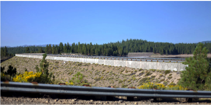
View of upstream face of Stampede Dam showing 11.5 foot high crest raise
