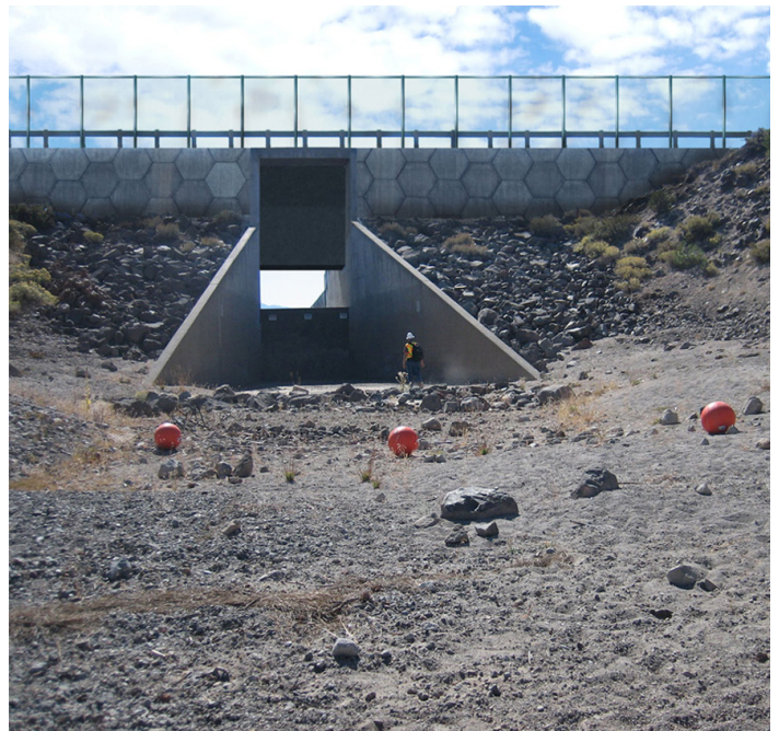
The spillway at Stampede Dam underwent significant modifications to enhance its capacity to handle extreme flood events
